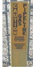
Example of a natural gas pipeline marker.
